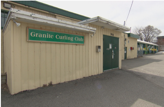
Figure 4.0 - Existing Granite Curling Club, 2026 Scott Street.
