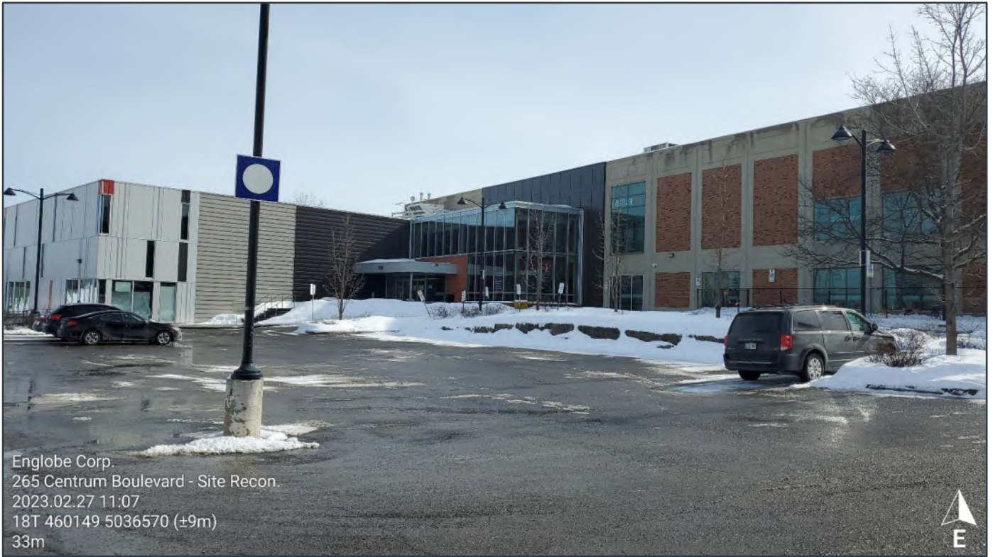
Site Photograph 1: Overview of the Entrance to the Site building (original build and new addition).
