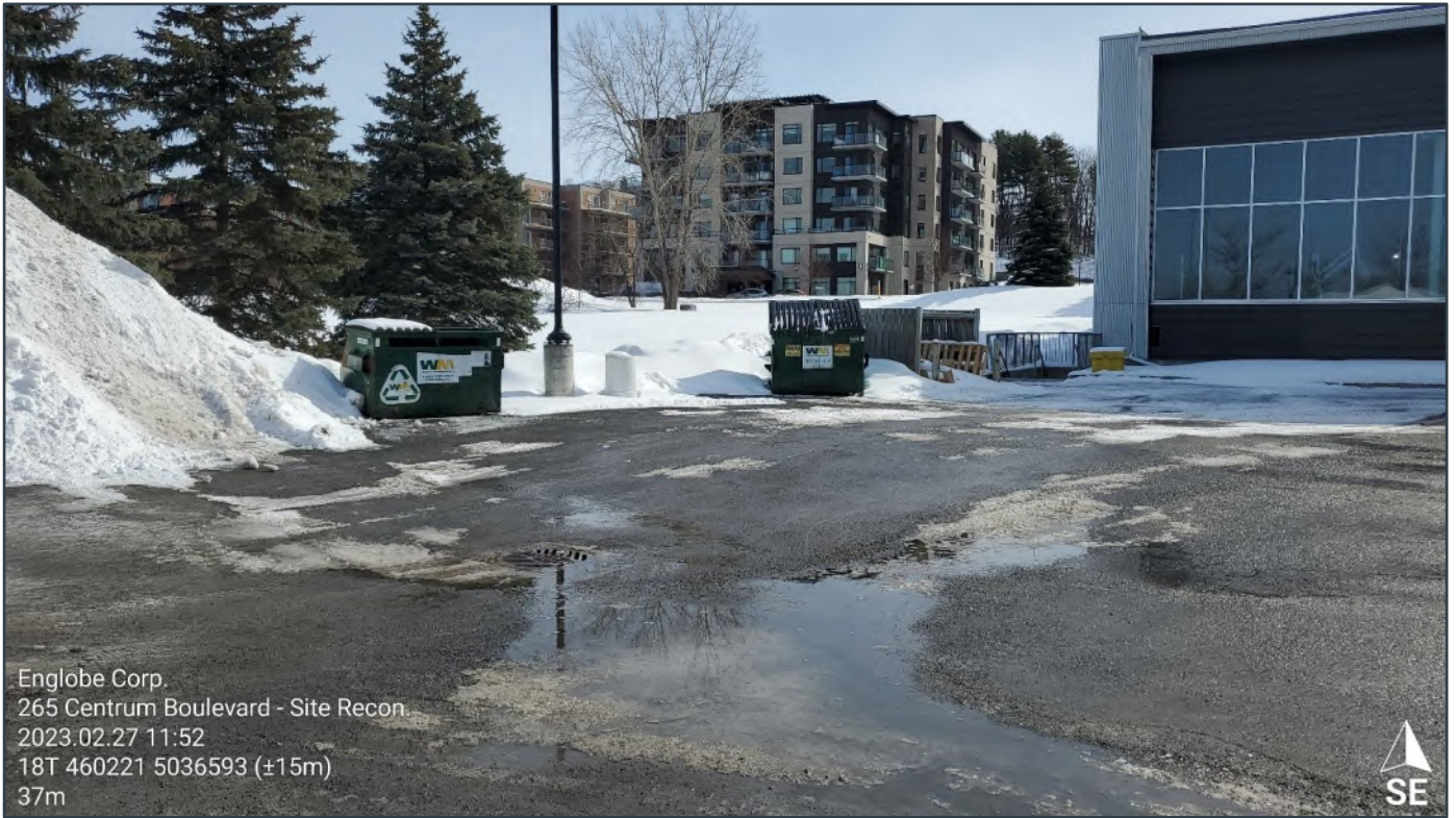
Site Photograph 3: Overview of the Site building (new addition) and waste collection areas.
