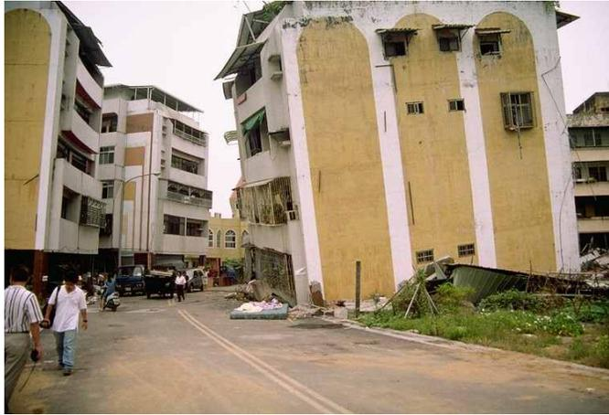
(a) 5- and 6-story buildings with foundation failures near the locations of borings WAS-3 and WAS-4 (photo by R. B. Seed)
