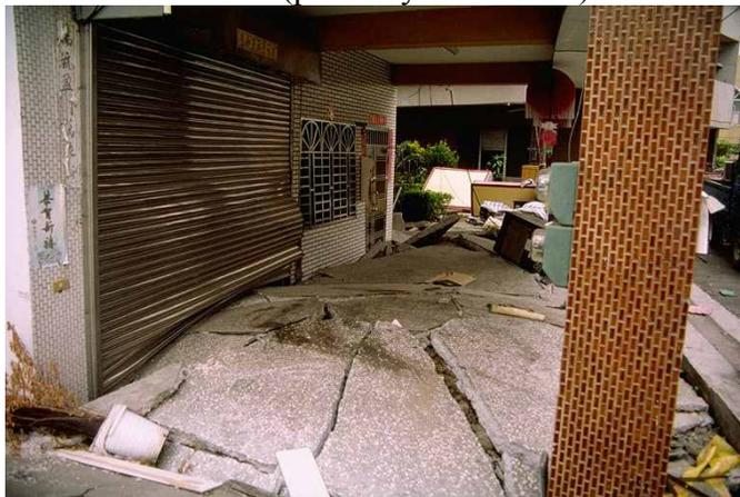
(c) Close-up view of foundation failures beneath a building [seen on left side of photo (a)] near the locations of borings WAS-3 and WAS-4 (photo by R. B. Seed)
