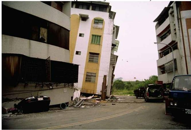
(b) 5- and 6-story buildings with foundation failures near the locations of borings WAS-3 and WAS-4 (photo by R. B. Seed)
