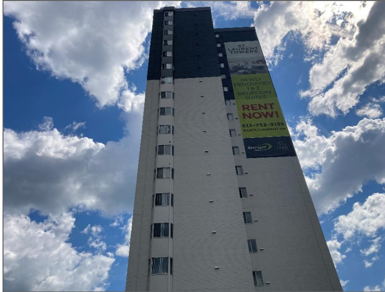
Photo 1 – Site Building A (northwest elevation).
