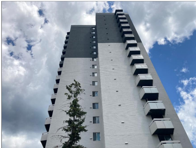
Photo 4 – Site Building B (southwest elevation).
