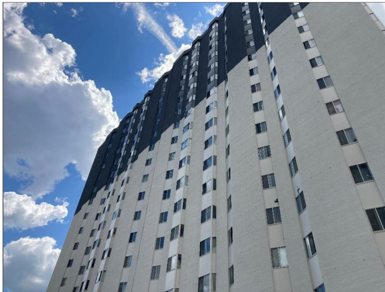
Photo 2 – Site Building A (northeast elevation).
