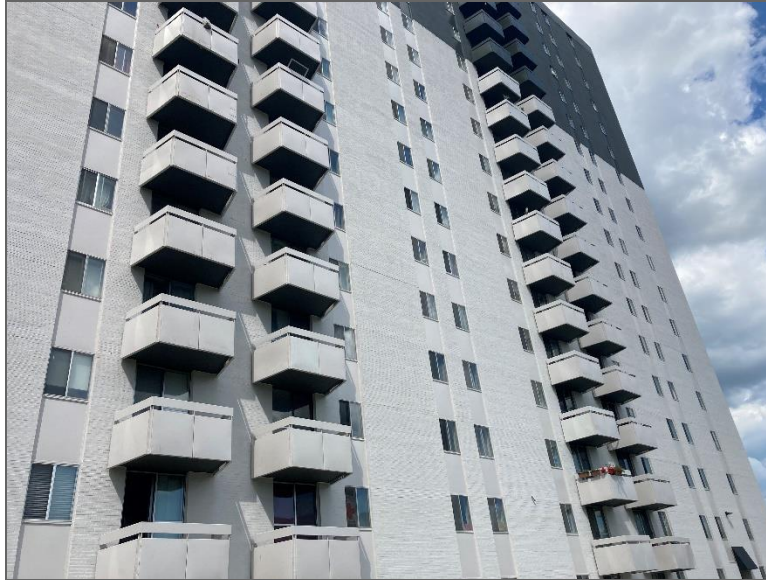
Photo 3 – Site Building B (southeast elevation).
