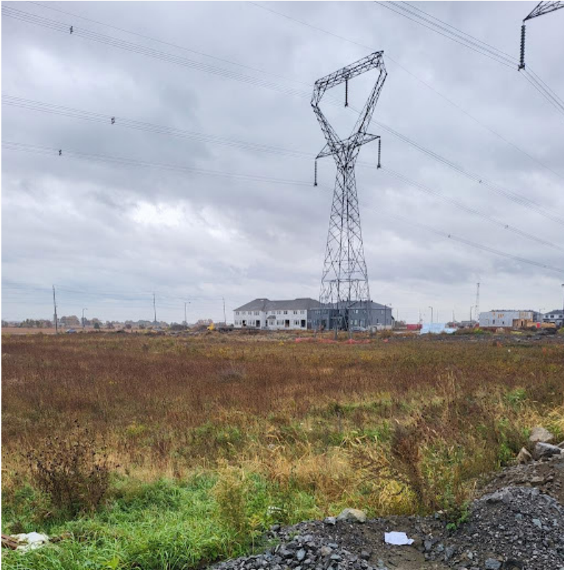
Photo #3 – Looking southeast across the hydro easement with the houses under construction on Cosanti Drive under construction.
