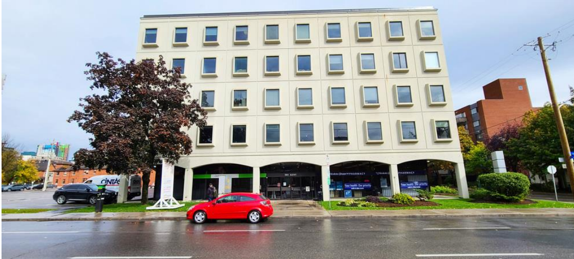
Figure 11: The view from Kent Street presents a façade identical to the other three sides with an arched arcade and the ground floor retail set back. The upper floors are a cream toned concrete with score lines defining each level and evenly spaced punched windows set-in a raised frame. Source: Google maps.
