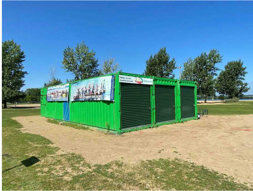
Photo 1: The sea cans (Site Buildings) occupied by the Petrie Island Canoe Club, located at 795 Trim Road, Orleans.
