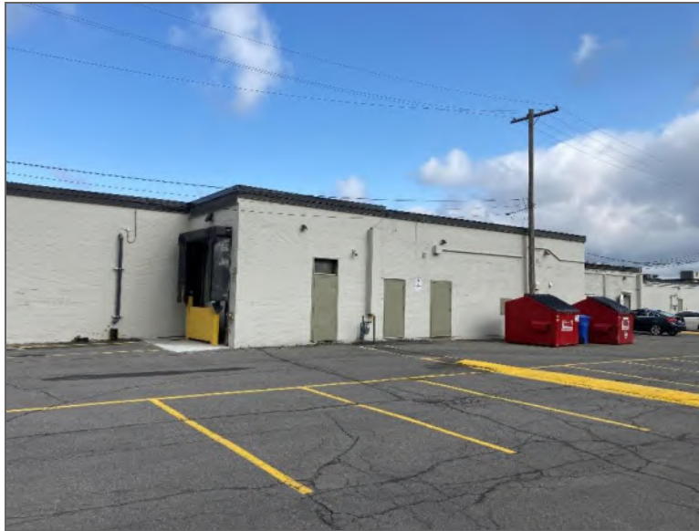
Photo 3 – Site Building (southeast elevation).
