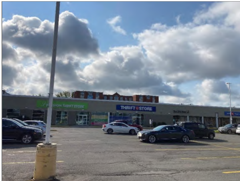
Photo 4 – Site Building (southwest elevation).
