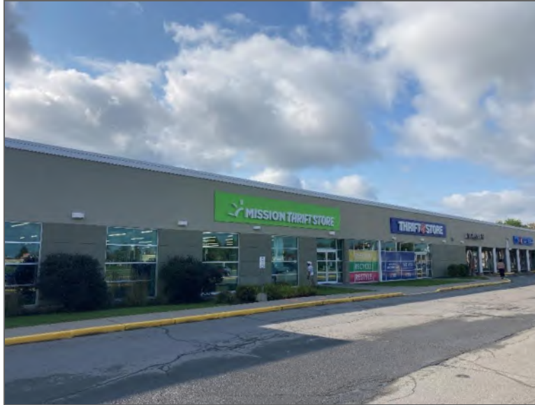
Photo 1 – Site Building (northwest elevation).
