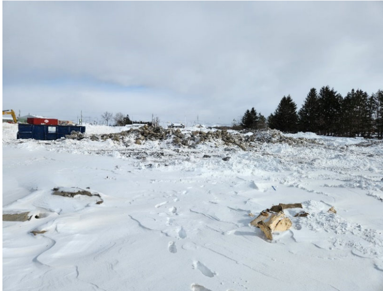
Photo 5 - Looking east, dumpster and aggregate piles
