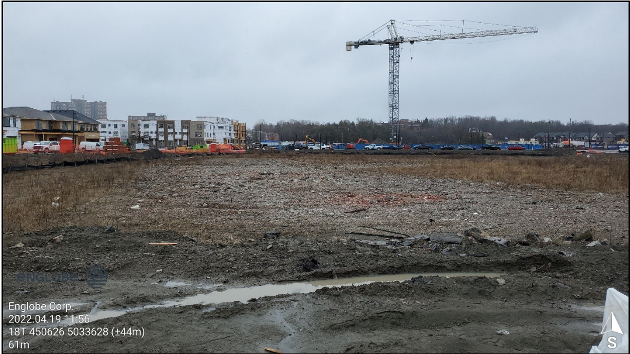
Photograph 1: View of Block 11 Parcel 1 facing south.
