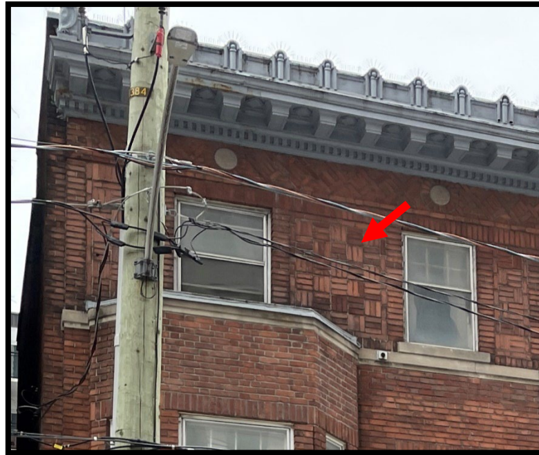
Figure 15: After the Wendell Apartments block was remodelled in 1941, the original facade disappeared behind an addition that likely contained a fire-resistant staircase. The remodelling reinstated or replaced the decorative cornice, but obscured and removed elements that contributed to a more recognizable Italianate style. One of these elements as the basket-weave brickwork (arrow). Source: Matrix Heritage, 2023.
