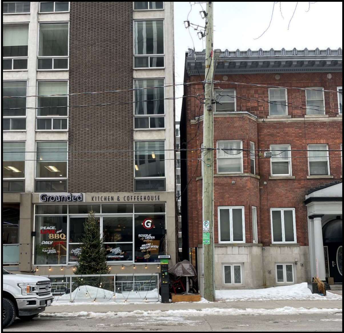
Figure 4: 100 Gloucester Street (left) and 110 Gloucester Street (right). (Credit: Matrix Heritage, 2023.)
