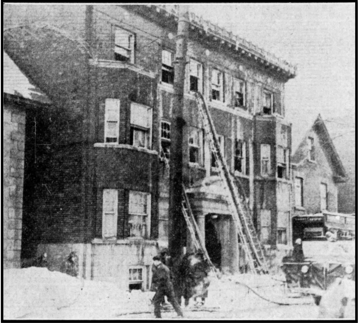
Figure 14: Wendell Apartments, 110 Gloucester Street, Ottawa, ON, after the fire in 1941. The quality of the image makes it difficult to fully discern its architecture, but it included a more fully articulated band below the attic storey and a shallow stone portico. Source: Ottawa Citizen , 4 March 1941, p. 1, accessed through Newspapers.com.
