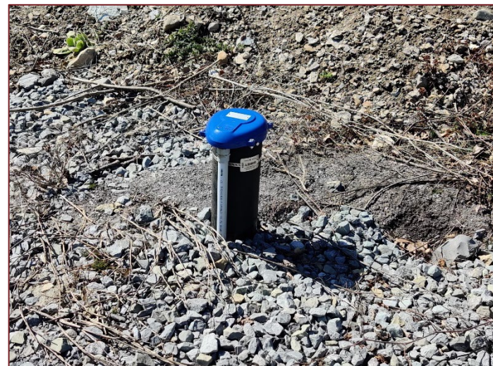
Photograph 6 – Potable well located west of the on-site office building near the northwest property boundary.
