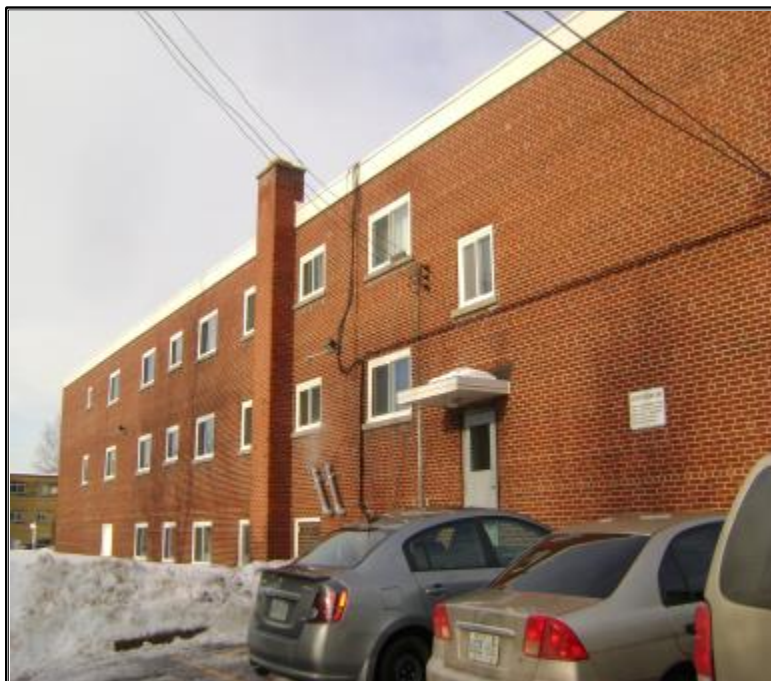
Photo 2 – General exterior view of the Site Building (south elevation).
