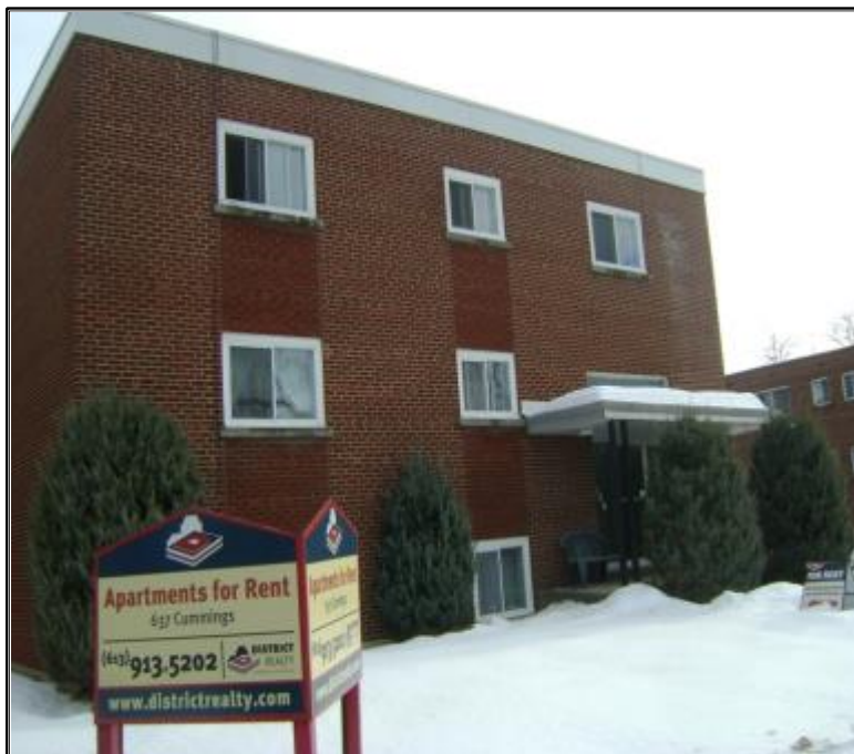
Photo 4 – General exterior view of the Site Building (west elevation).
