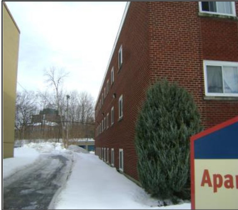
Photo 1 – General exterior view of the Site Building (north elevation).
