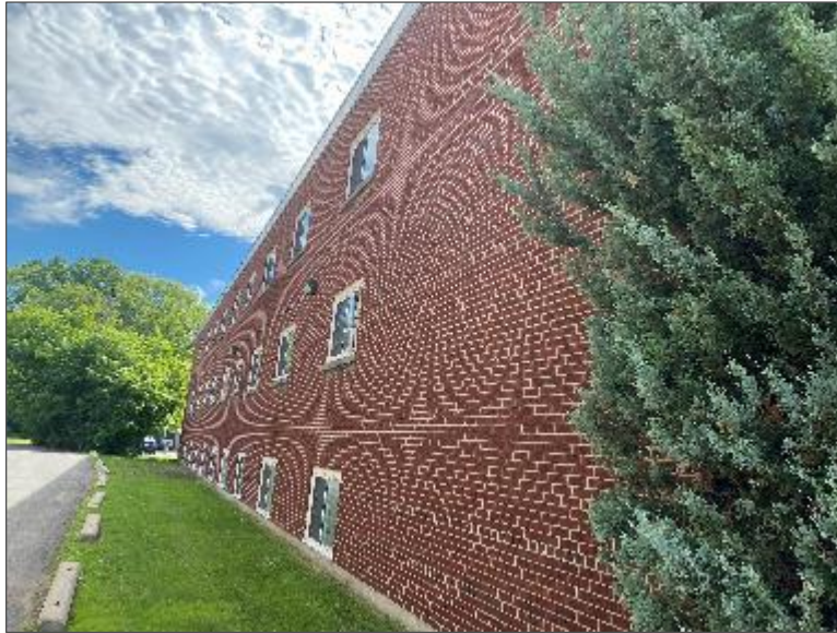
Photo 1 – Site Building (north elevation).
