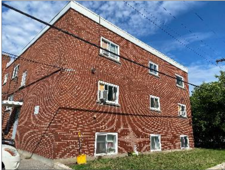
Photo 3 – Site Building (east elevation).
