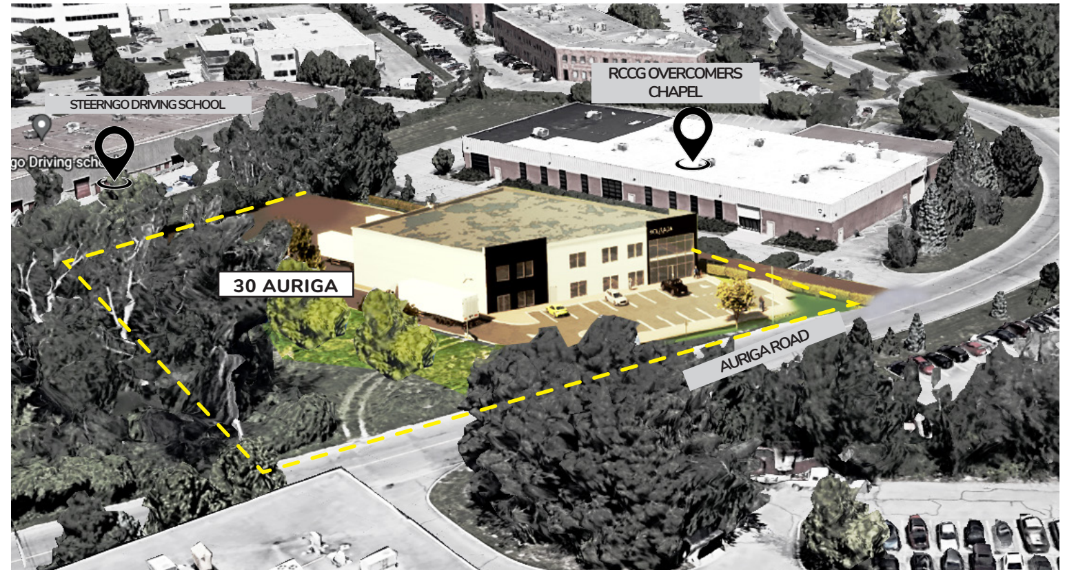
4 - AERIAL VIEW FROM SOUTH EAST TO NORTH EAST
