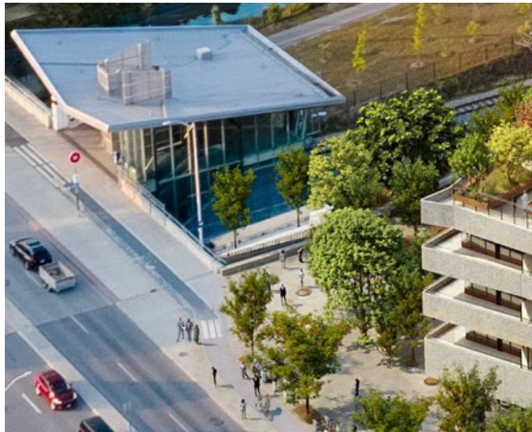
Figure 1 West Site access after the removal of parapet (2022-11-09)
