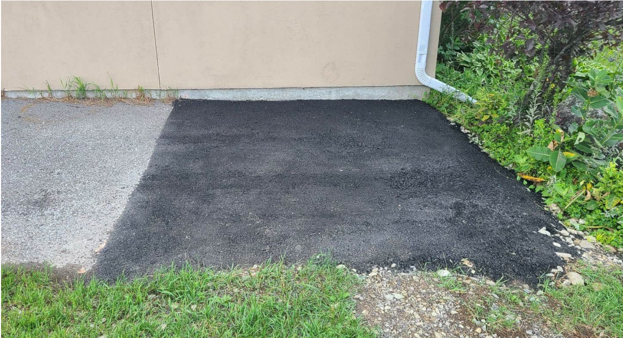
Photograph No. 4: Reinstated pavement conditions at Test Pit No. 1 location
