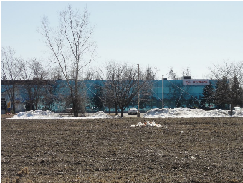
Photo 12 – View of commercial office buildings located adjacent south of the Site, looking southwest.
