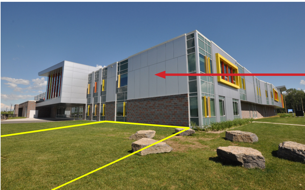
PHOTOGRAPH 08 View of north facade at proposed Addition Existing composite aluminum panels removed for the construction of the Addition will be re-used on the west facade of the Addition.
