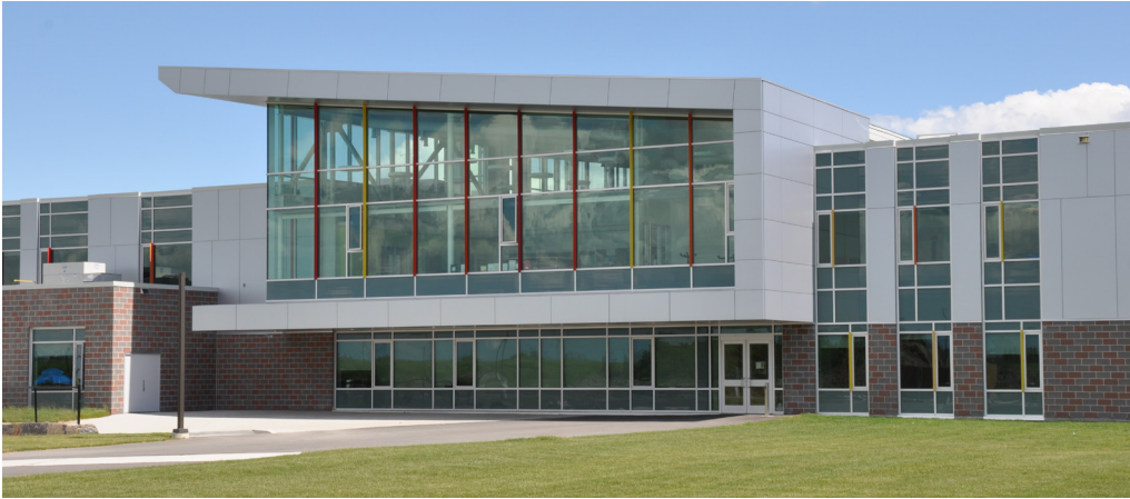
PHOTOGRAPH 06 View of north facade entrance serving parking lot
