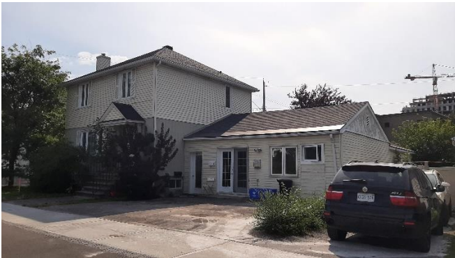
Figure 1: Existing dwelling viewed from the northwest on Scott Street, with the two (2) storey dwelling shown on the left and the one (1) storey addition shown on the right
