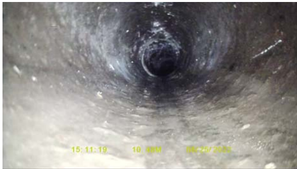
Figure#7: A view to the roots fine from 9 to 4 o'clock at 13 meters from the top of Back Water Valve (BWV).
