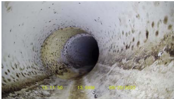
Figure#11: A view to the right line deviation at 15.8 meters from the top of Back Water Valve (BWV).
