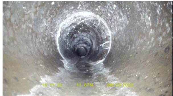
Figure#8: A view to the material change to PVC at 13.2 meters from the top of Back Water Valve (BWV).
