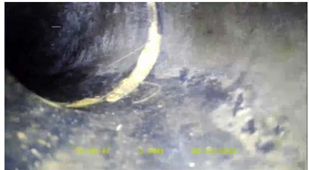
Figure#4: A view to the line deviation downwards at 9.6 meters from the top of Back Water Valve (BWV).
