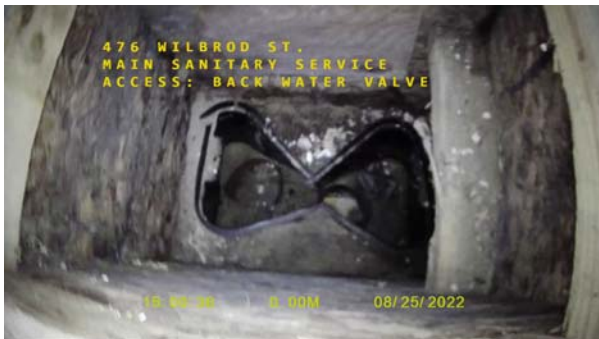
Figure#3: A view to the right line deviation at 1.4 meters from the top of Back Water Valve (BWV).
