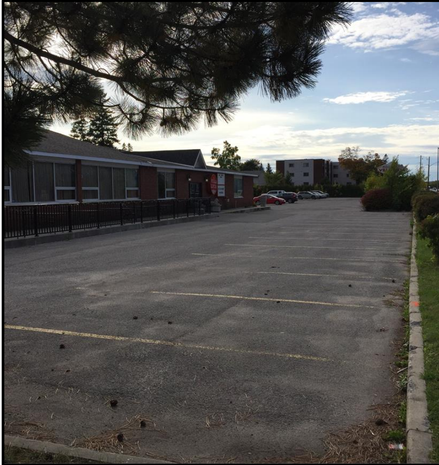
Photograph 3: View of the Phase I Property, taken from the east of the site, looking west.
