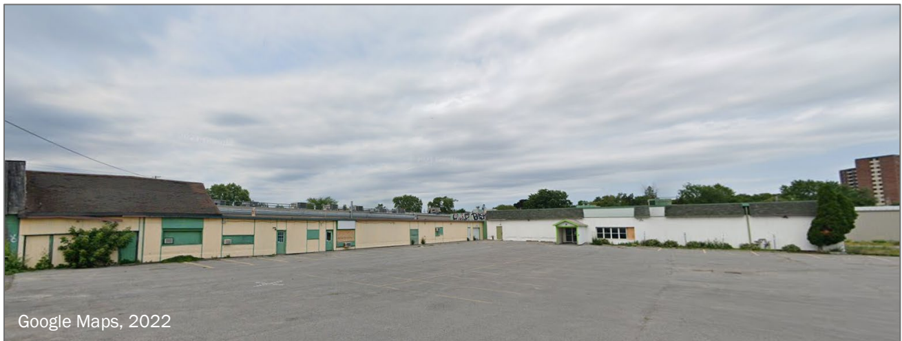
Figure 4: View from front of site looking north on Merivale Road
