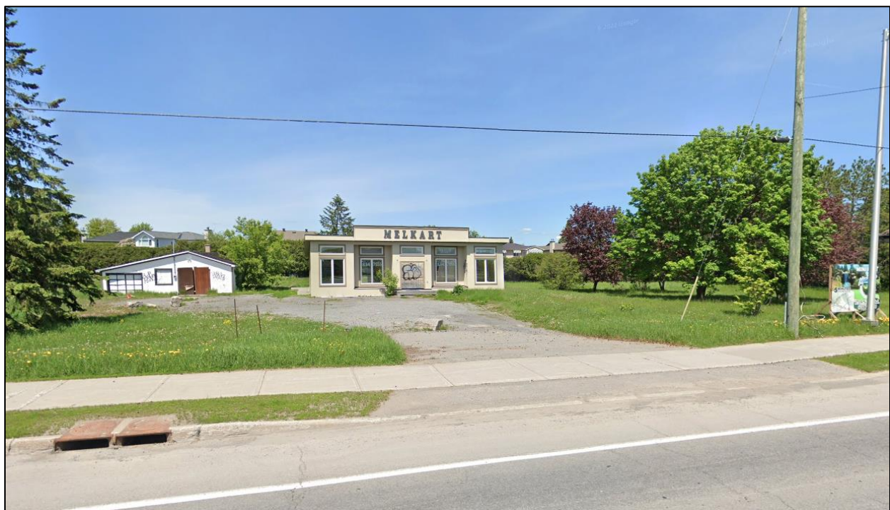
Figure 2: Existing Conditions on the subject site (note: buildings have since been removed).
