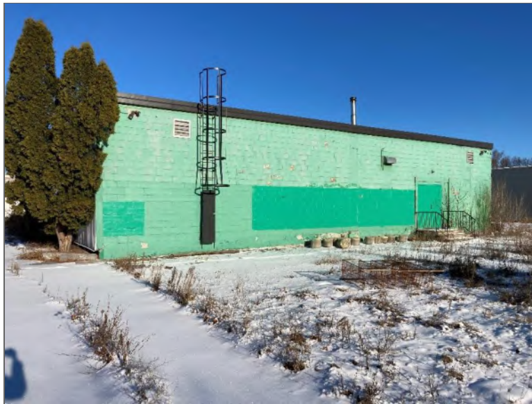
Photo 2 – Site Building B (south elevation).
