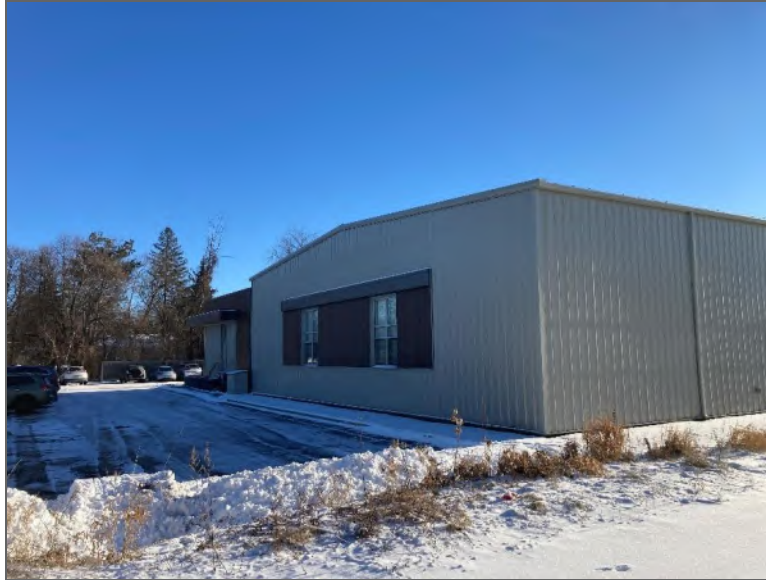
Photo 7 – Property located east of the Phase One Property.
