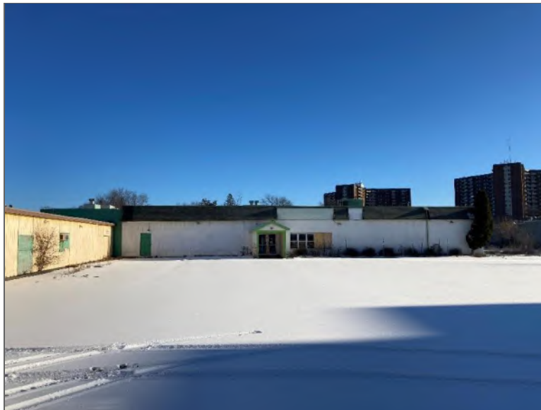
Photo 4 – Site Building B (west elevation).
