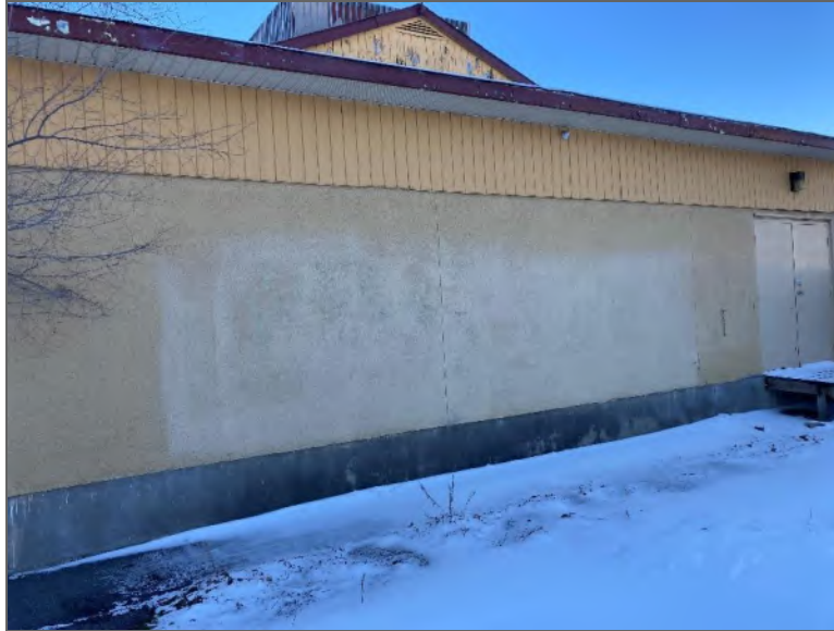
Photo 3 – Site Building A (east elevation).
