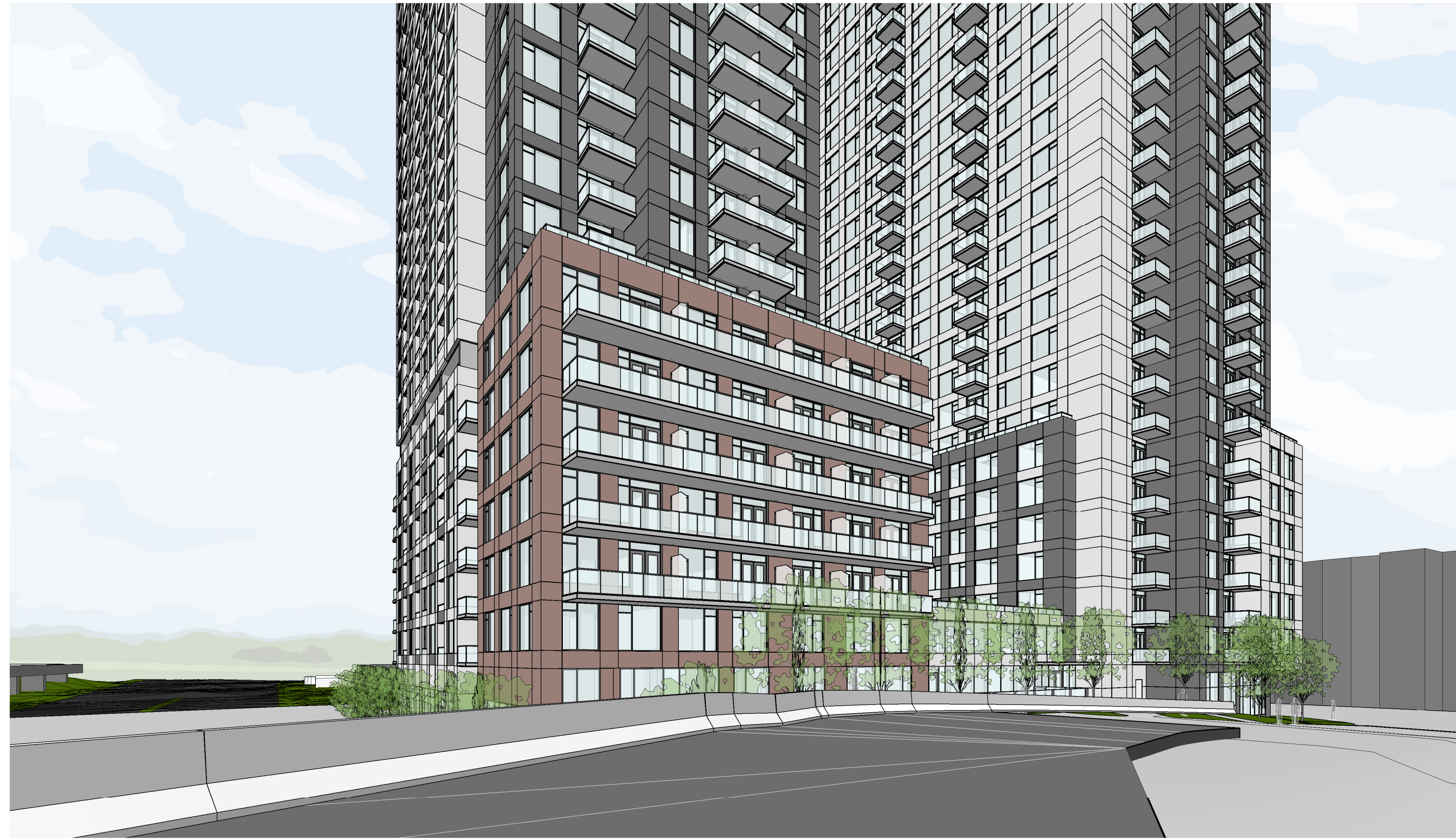
VIEW NORTH-EAST OVER BRIDGE
