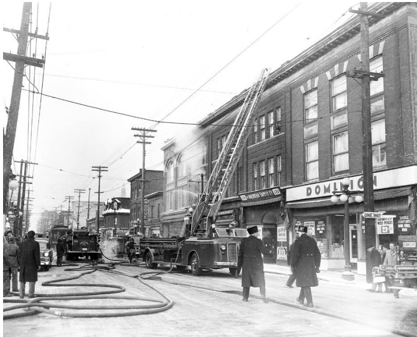
Figure 24: This c1950 street view looking north with the firetrucks in the street provides guidance for the reinterpretation of shopfronts. Source City of Ottawa Archives. The view below has been photoshopped and the shopfronts interpreted.
