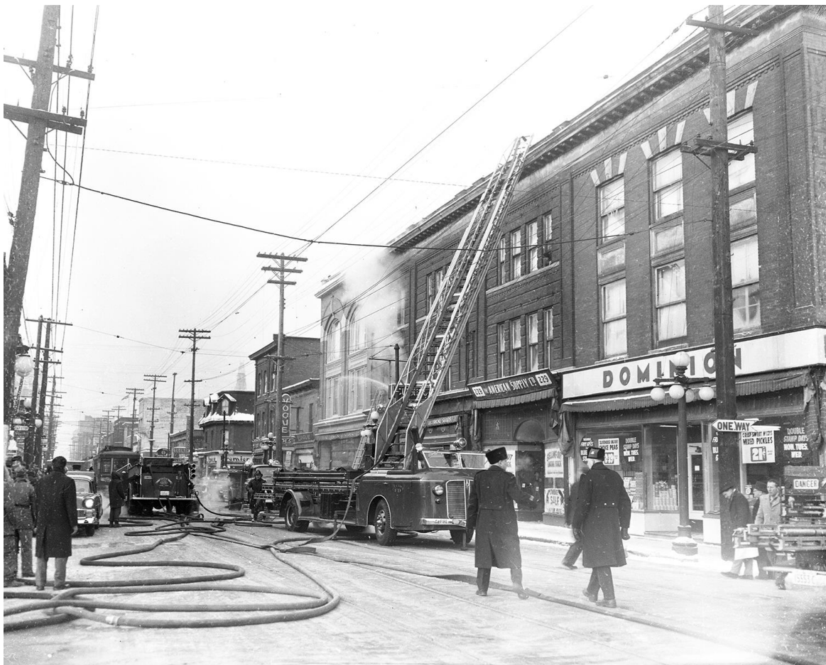
Figure 17: A view of the 211-231 block with fire trucks in the street. Note the unpainted facades with the decorative keystone with spandrels between the 2 nd and 3 rd floors. The photo provides a record of the earlier retail storefronts.
