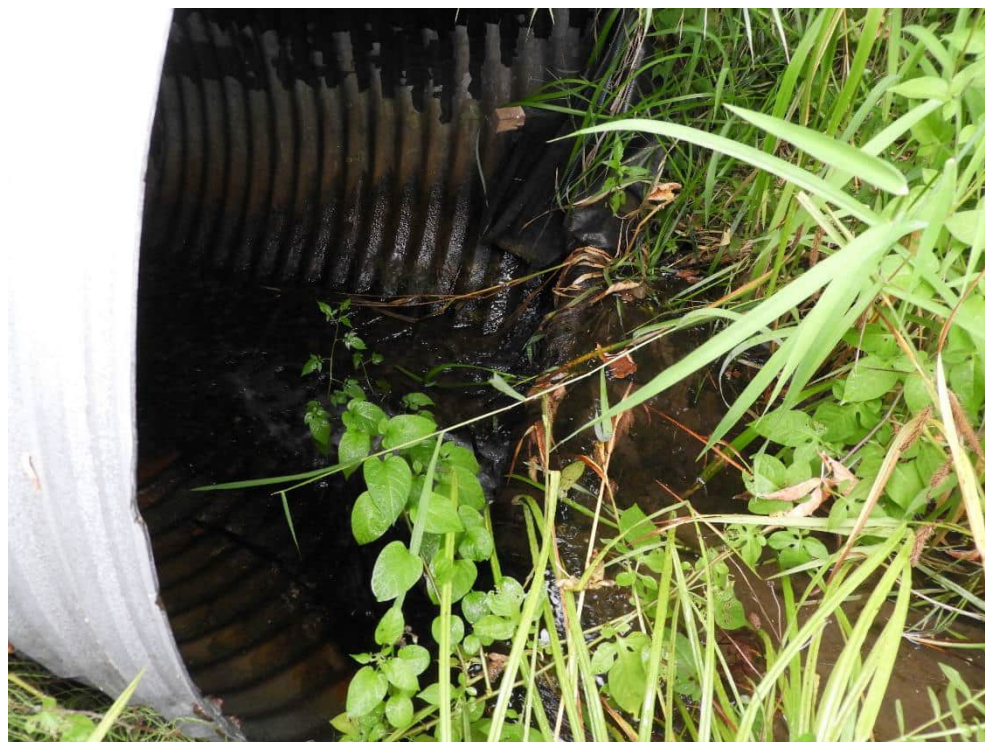
Photo 8: View of inlet of the culvert under Russ Bradley Road which conveys the tributary of Carp River from inside the study area to outside the study area. 11 August 2021.
