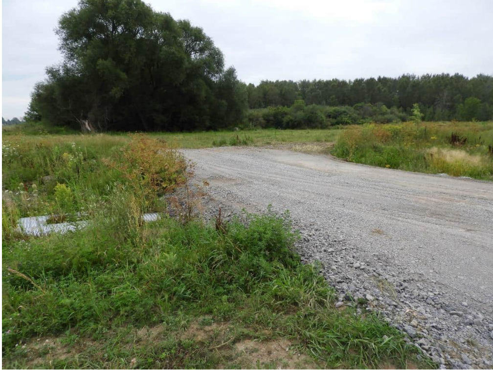
Photo 5: Constructed entrance with twin culverts from Russ Bradley Road over the realigned tributary of Carp River in the west end of the Forb Meadow. 11 August 2021.
