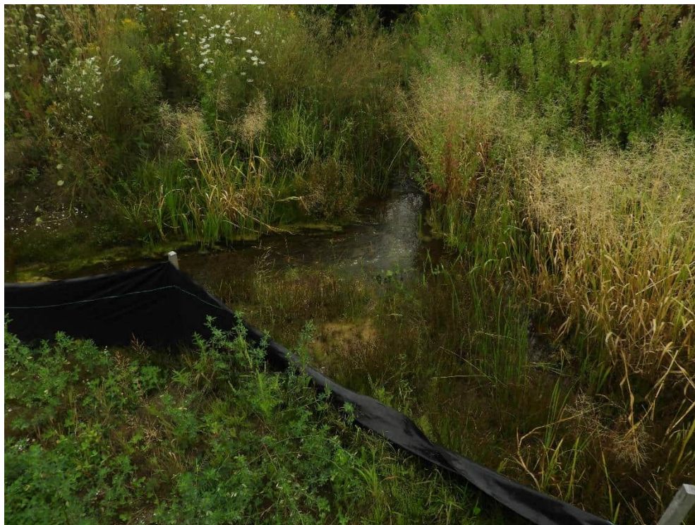
Photo 7: Ditch line flowing northwest along the west side of Carp Road (right) draining into the tributary of Carp River flowing northeast along the south side of Russ Bradley Road (left). The confluence then flows northwest under Russ Bradley Road (top). 11 August 2021.
