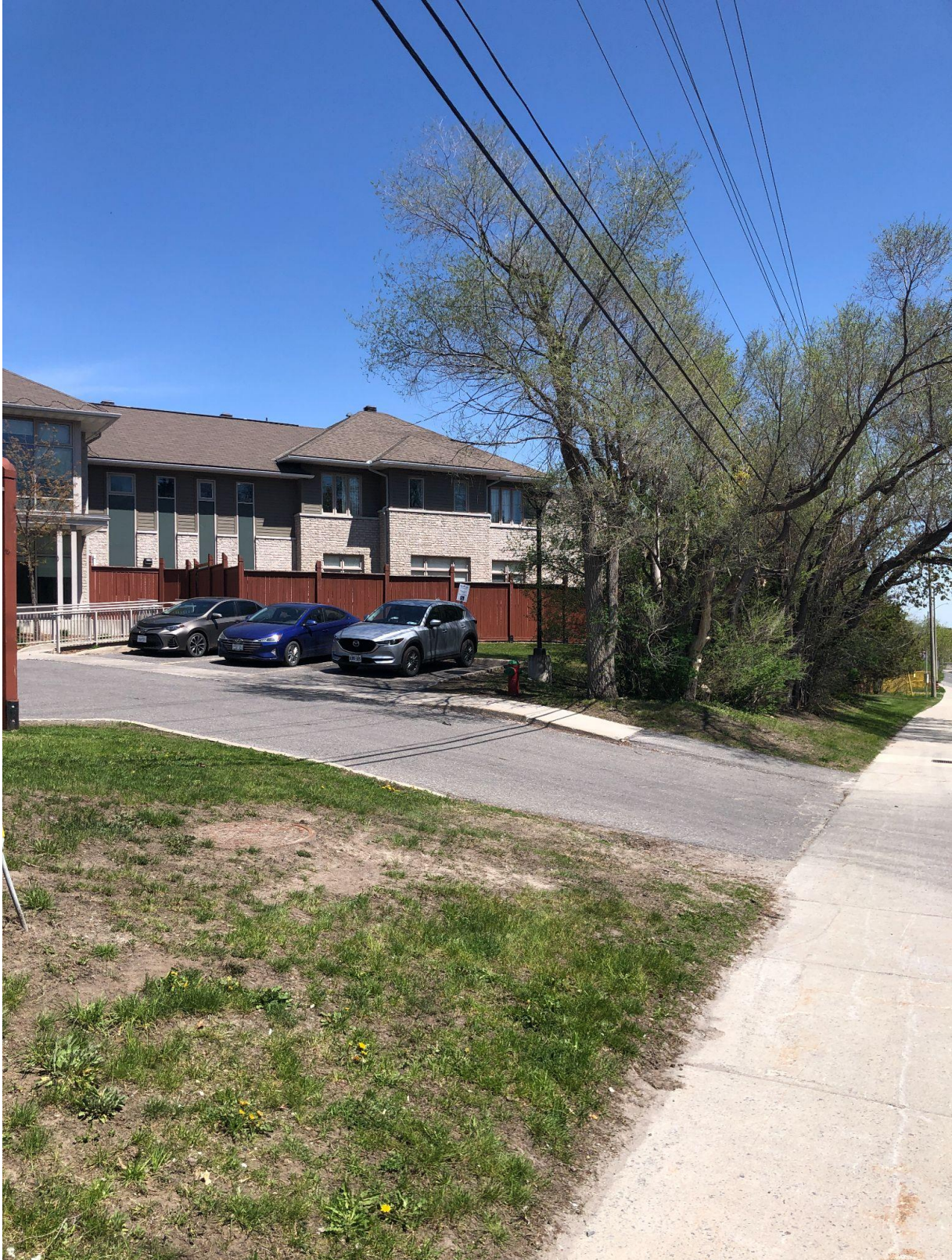
1777 Montreal Rd. (Montfort Residence) east of 1765 Montreal Rd. View looking east.
