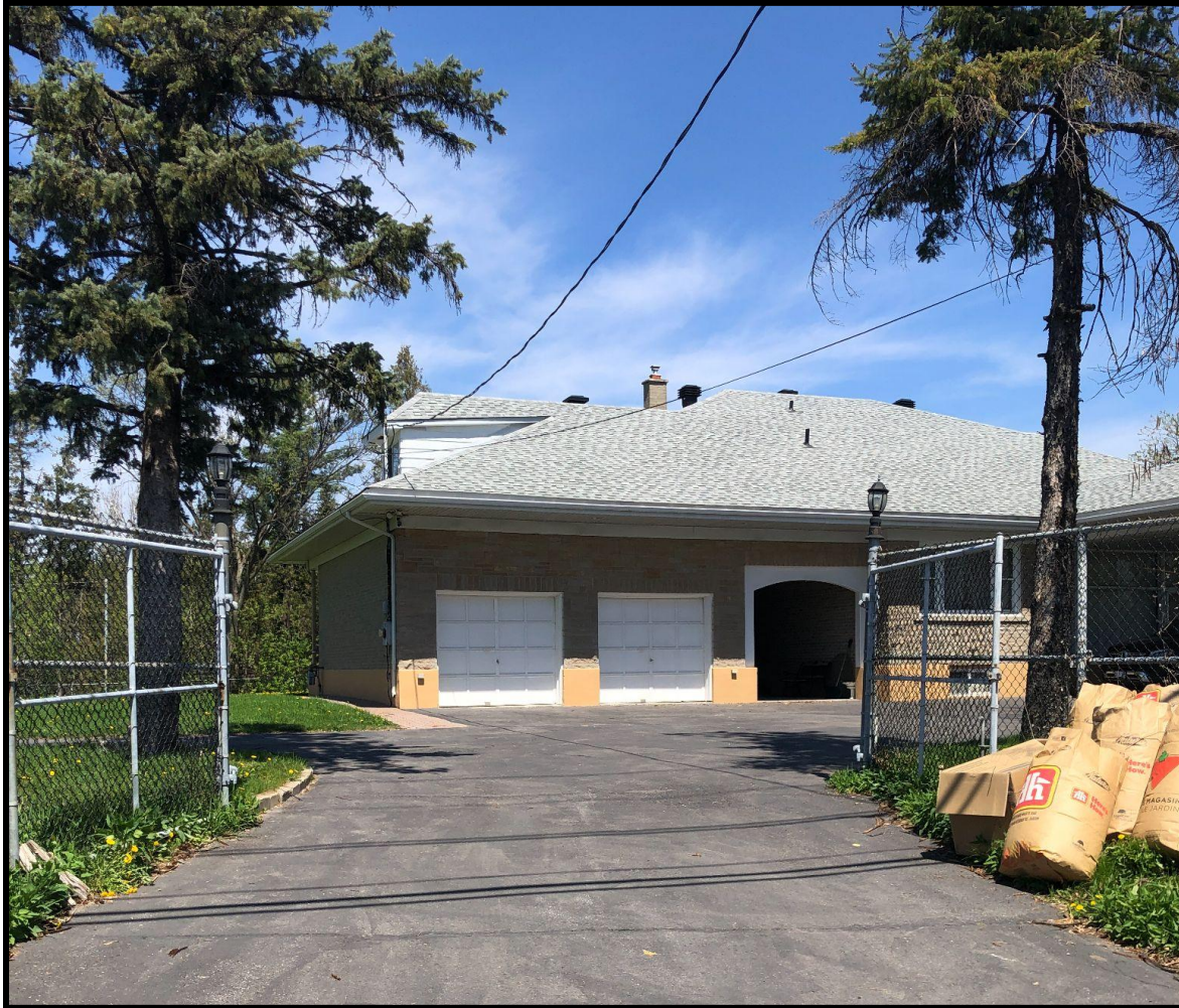
Existing building (front facade) at 1765 Montreal Rd.
