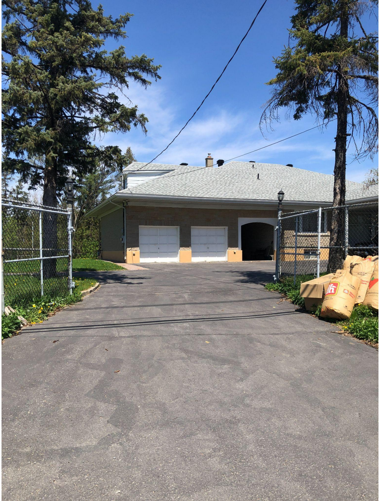
Existing building (front facade) at 1765 Montreal Rd.
