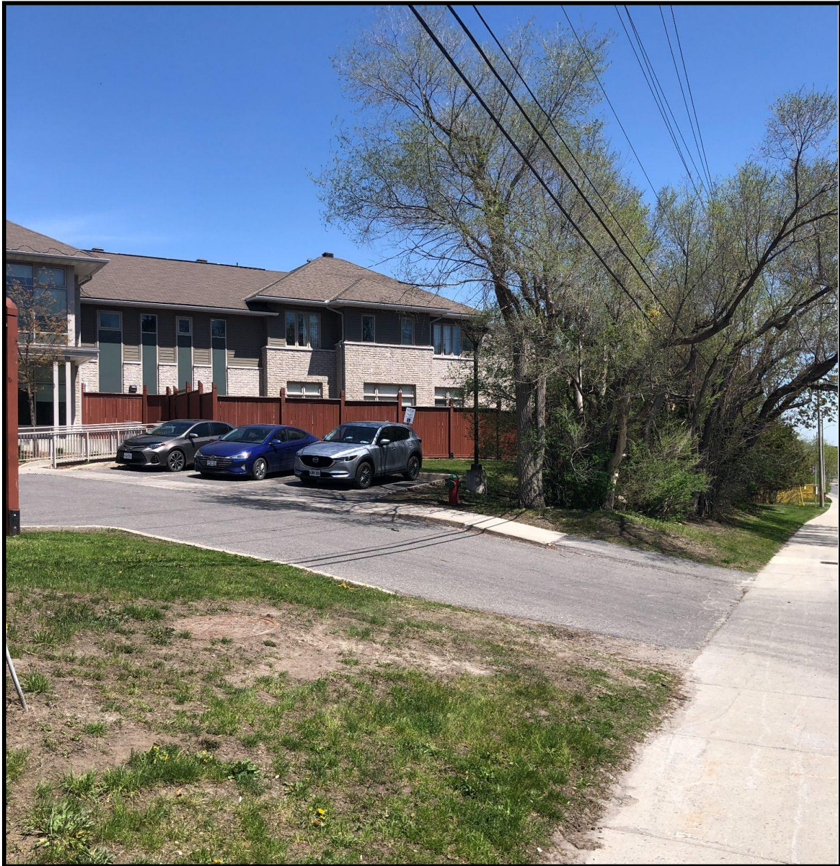
1777 Montreal Rd. (Montfort Residence) east of 1765 Montreal Rd. View looking east.
