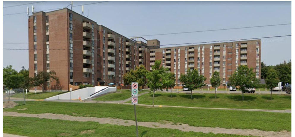
Photo 7: Innes Park Complex
