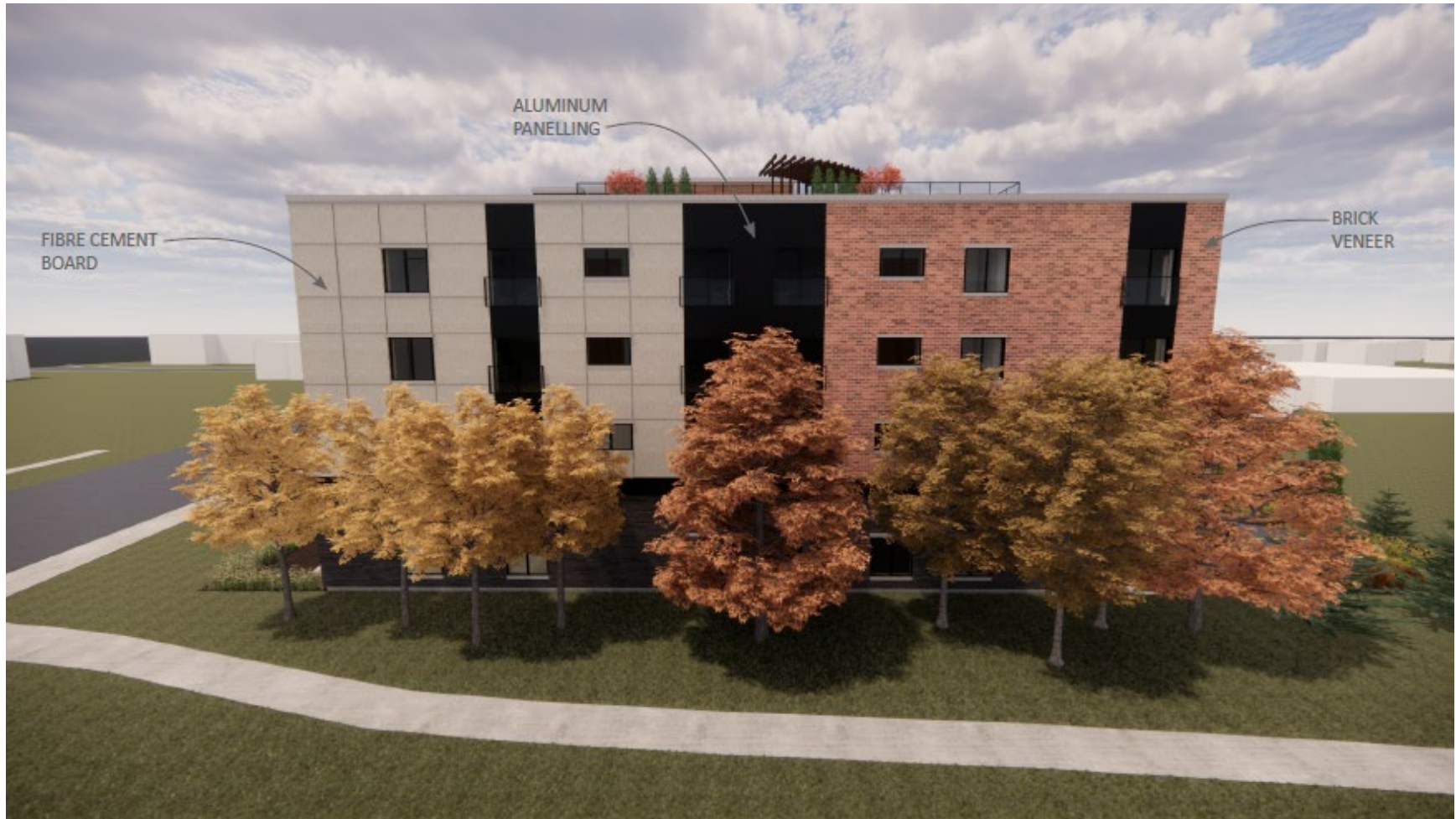
Figure 6 - East facade at walking path to Bearbrook Park
