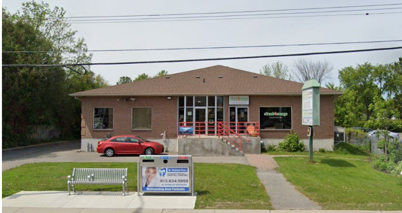
Photo 14: Commercial Multi-Office space abutting Innes Road
