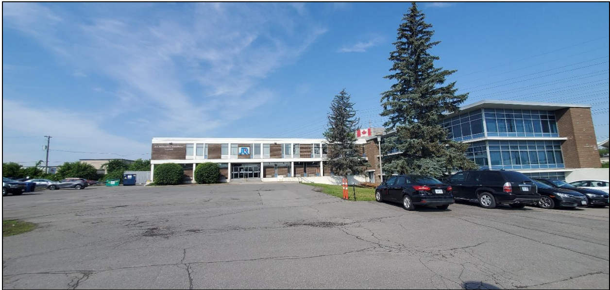
Figure 2-2: Existing three-storey commercial office building at 864 Lady Ellen Place
