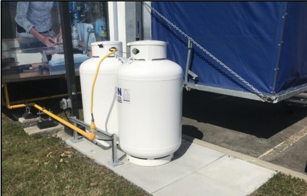
Photo 31: Photo of propane cylinders stored vertically on a concrete pad, to the south of the Site property.
