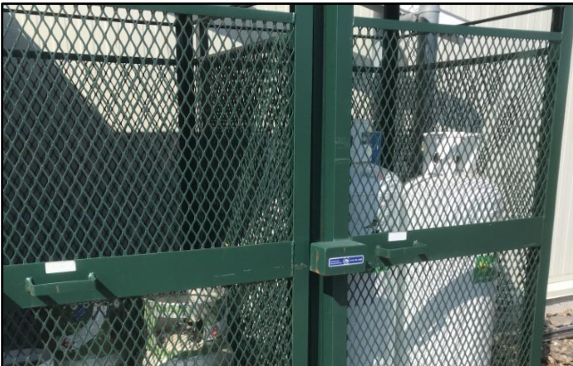
*Photo 28: Photo of propane cylinders secured vertically in a storage cabinet to the east of the Site building.*
