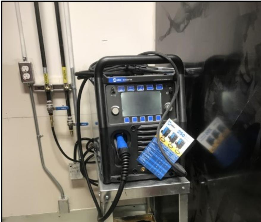
Photo 17: Individual workspace for welding training with argon piping.
