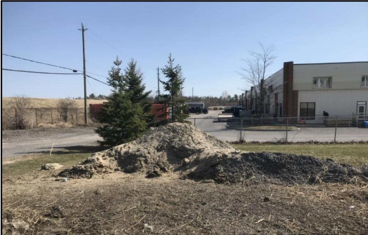
*Photo 25: Imported sand and gravel fill piles observed towards the northeastern corner of the Site.*
