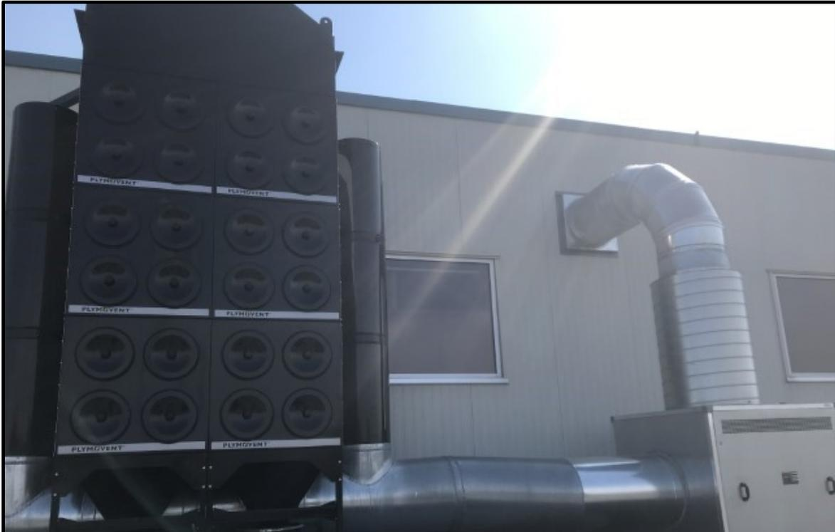
Photo 19: Central extraction fan with two drums for the collection of welding dust.
