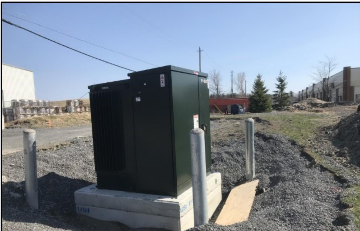
*Photo 26: Pad-mounted transformer located on the north-boundary of the Site.*
