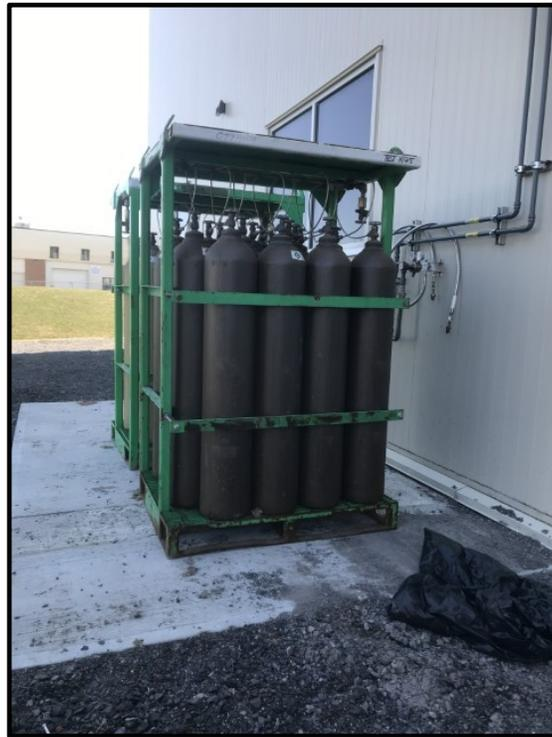
Photo 29: Photo of compressed argon cylinders secured vertically in two storage cabinets on a concrete pad, to the north of the Site building.
