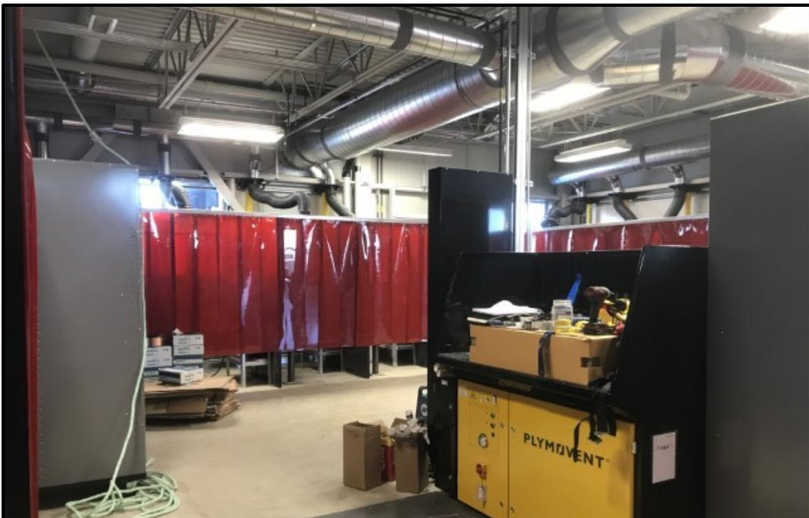
Photo 16: Welding training area with central extraction fan unit.
