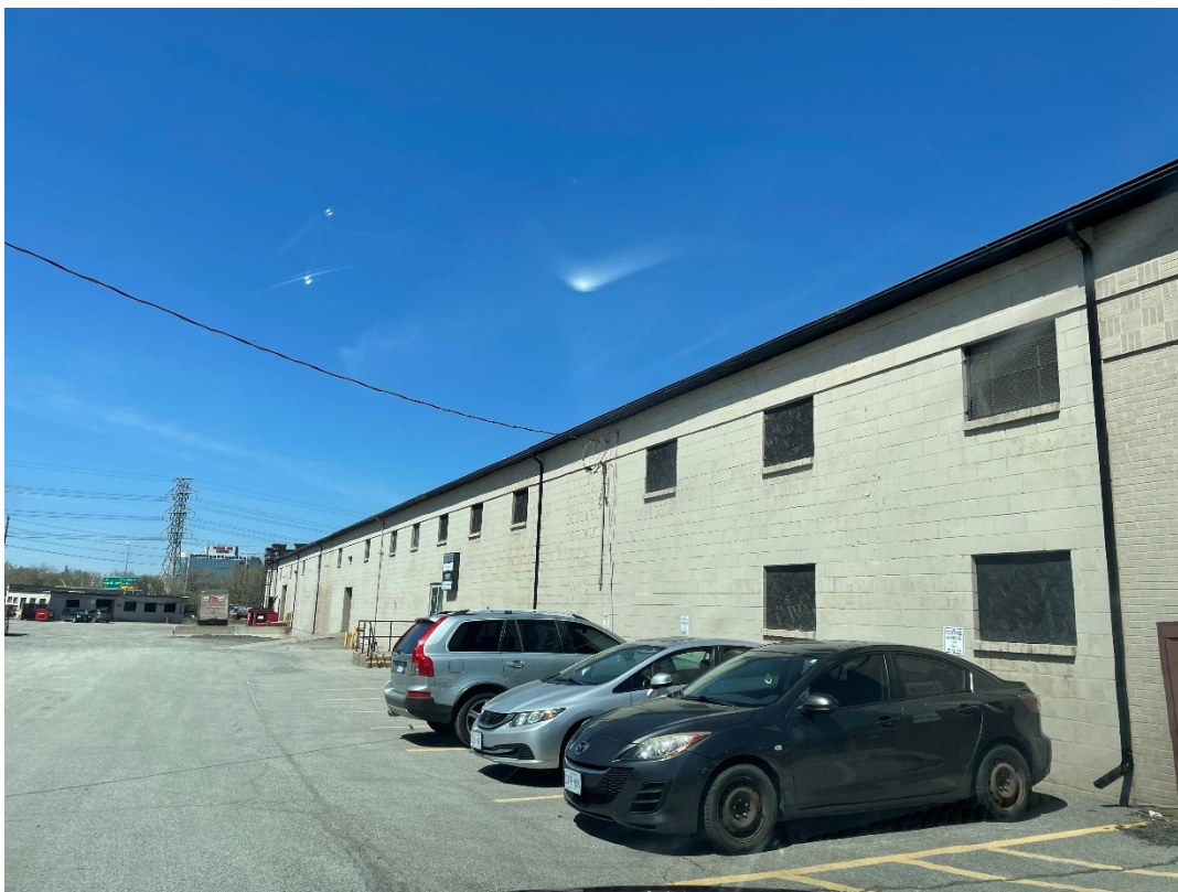
Photo 369: 1519 Laperriere Ave - Former tucker transport and chemical industry locations
