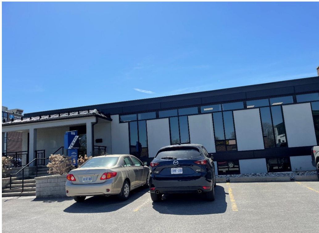
Photo 30: 1550 Carling Avenue (frontside) - Location of former activities including cosmetics manufacturing, commercial printing, and a diesel generator
