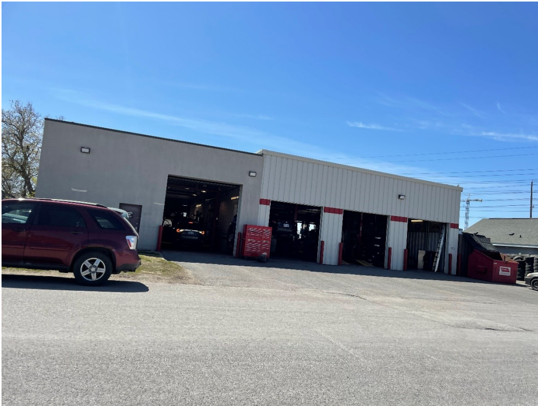
Photo 373: 895 Churchill Ave - Former and current auto service garage
