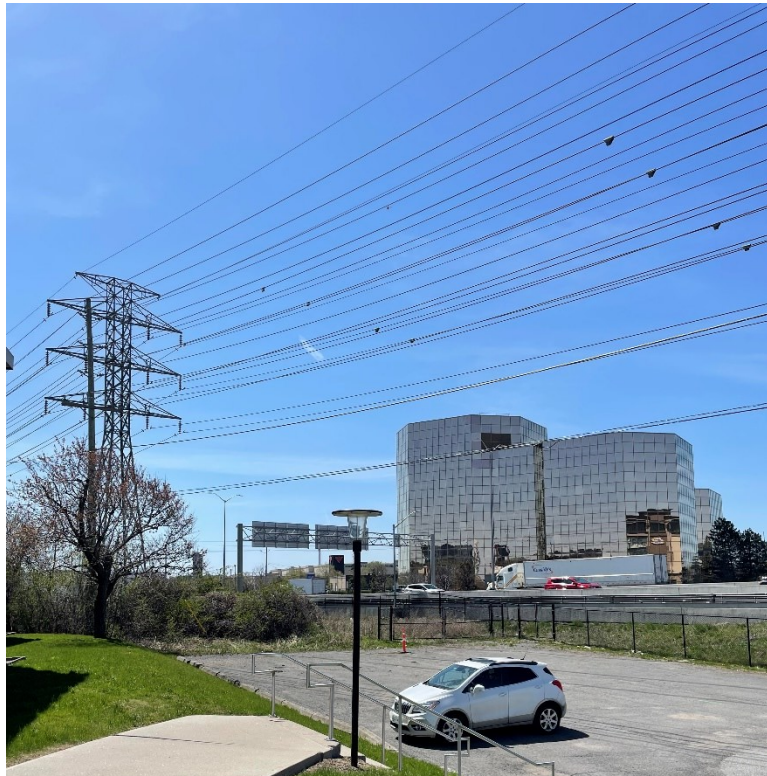
Photo 243: View from north of the building including electrical lines and the highway
