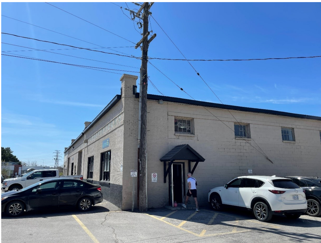
Photo 370: 1529 Laperrier Ave - Former manufacturing location
