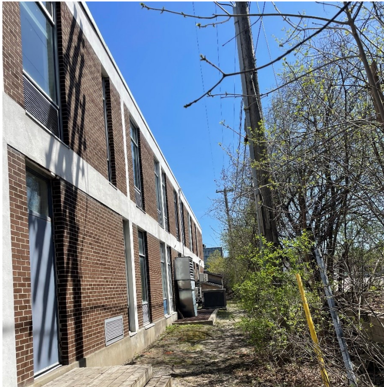
Photo 245: Other outdoor mechanical equipment
