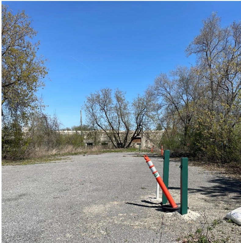
Photo 7: Stick up wells located in eastern parking lot
