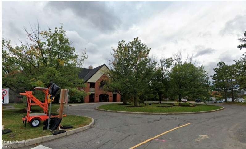
Photo 9: Existing House from the Street
