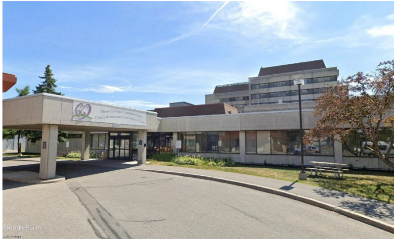
Photo 17: Ottawa Children's Treatment Centre Entrance
