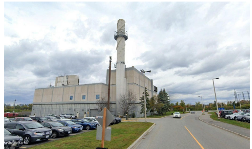
Photo 12: Trans Alta Cogeneration Plant
