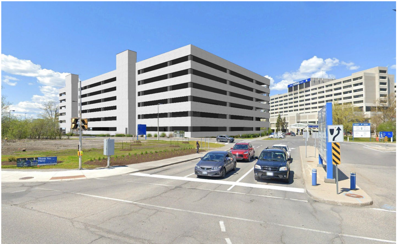
Figure 09 - Pedestrian Perspective, view from southeast (south side of Smyth Rd) - Google Earth context
