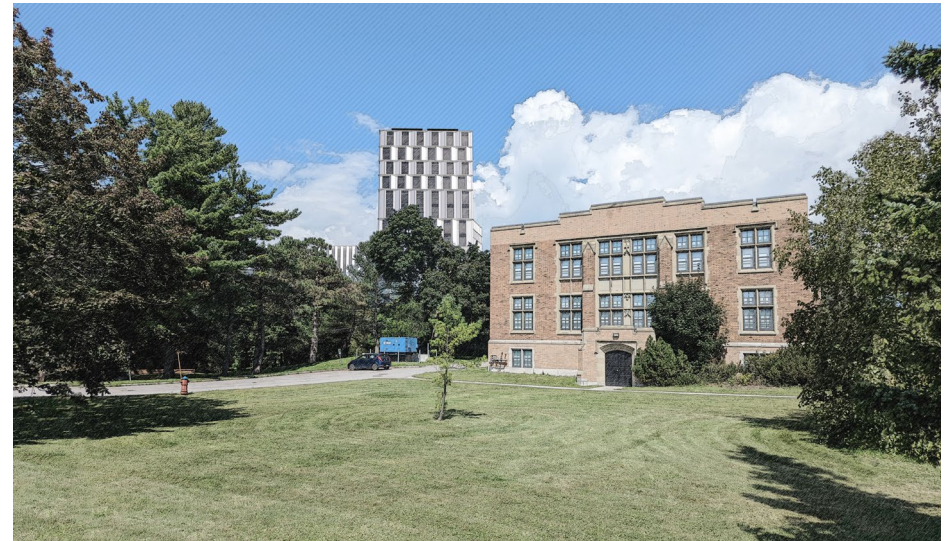
Figure 87: Views Analysis - Referenced Views #8 View from adjacent to the Saunders Building looking north - Tower B appears from behind the existing mature tree cover with the podium extending westward behind the existing tree cover.
