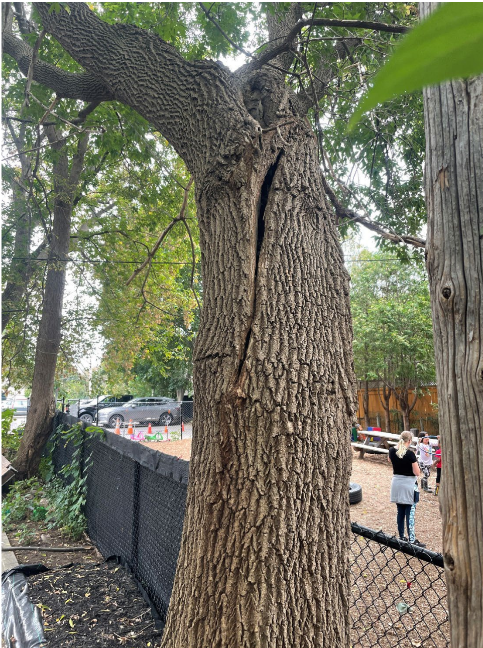
Figure 3: Vertical and horizontal stress fractures of tree 2 located on the upper side of the bend in the trunk
