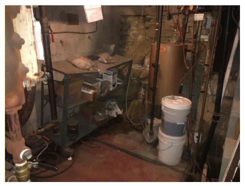
Photograph 29: Boiler blow down tanks in basement of Site building (April 6, 2021).
