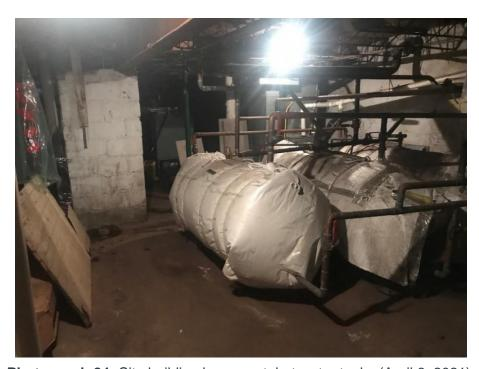
Photograph 24: Site building basement, hot water tanks (April 6, 2021).
