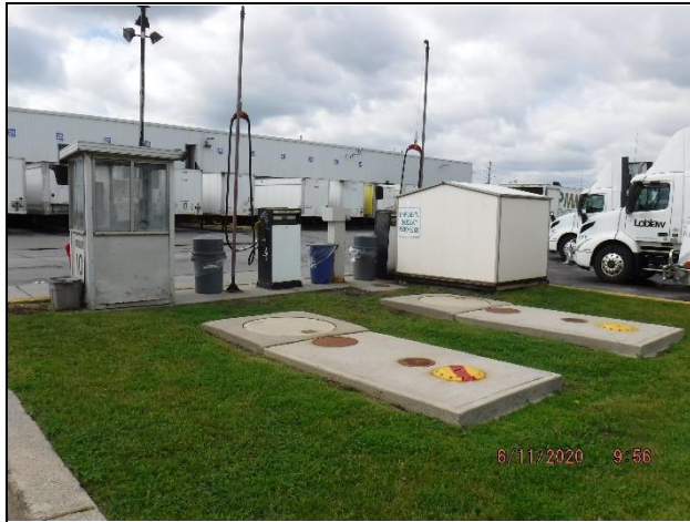
Photo 1: Existing Fuel Station
