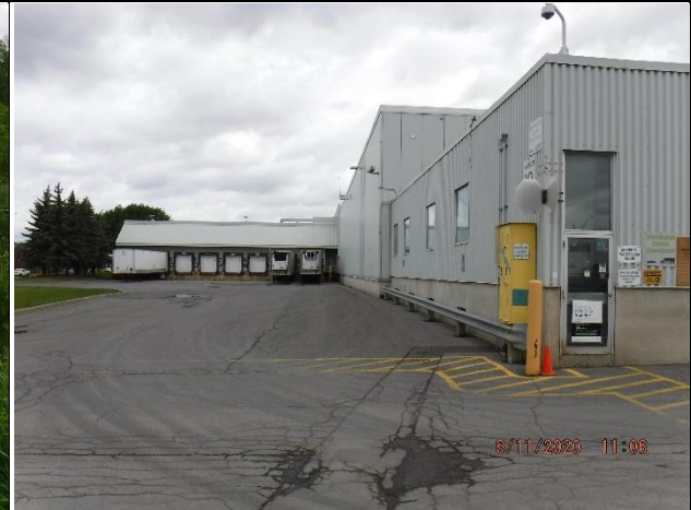
Photo 8: Existing Parking Lot
