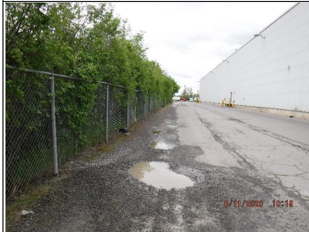
Photo 5: Existing Site Perimeter Fence
