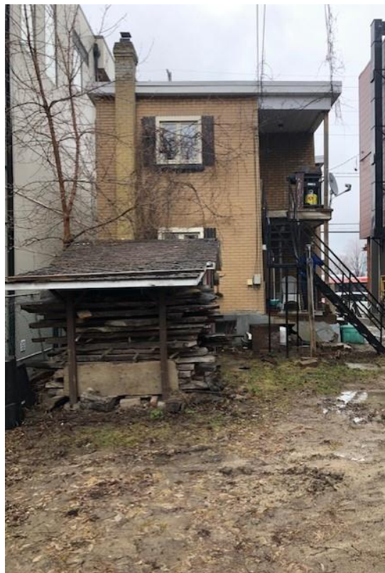
Photograph 2: View of the western portion of the subject site, facing east.
