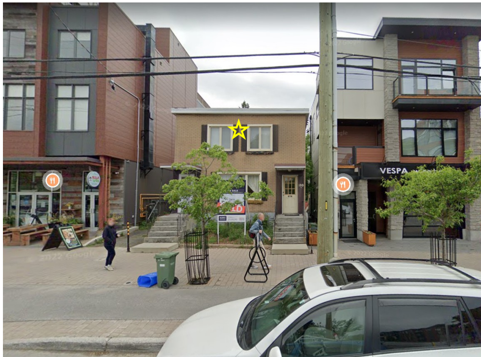
Image 6.1 – view from the street looking at the existing building at 180 Main St.
