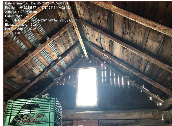
Site Photograph 4 – Barn Interior
