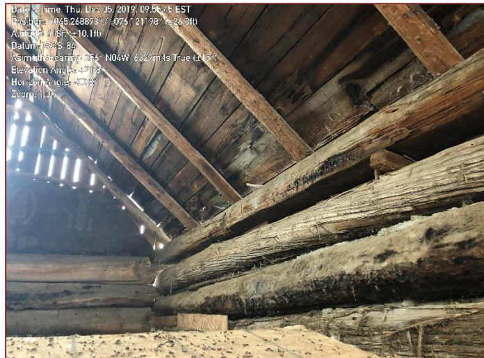
Site Photograph 3 – Barn Interior
