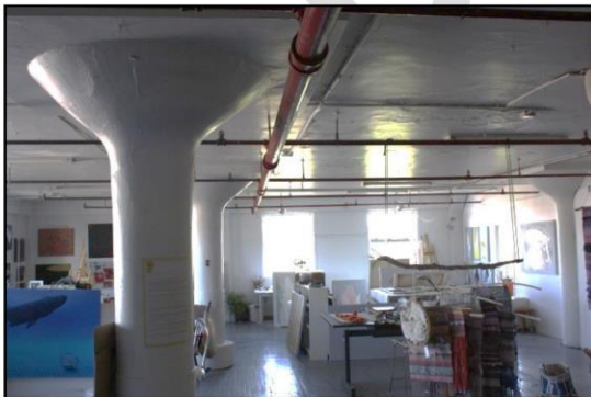
Photo 2: Typical columns inside the building [JCAL 2018].
