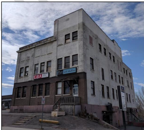
Photo 1: 951 Gladstone Avenue, south and east elevations [JCAL 2018].
