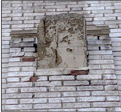
Photo 4: Typical corbel on the west elevation. Concrete and bricks are deteriorating [JCAL 2018].
