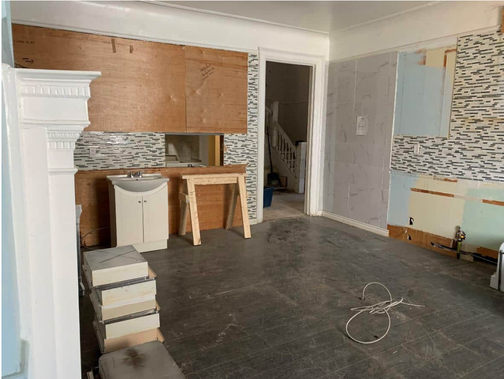
Photo 1: Living area on the ground level of the Site Building.
