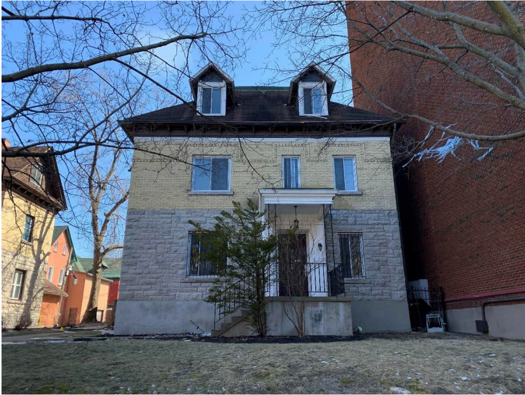
Photo 9: North exterior of the Site Building.
