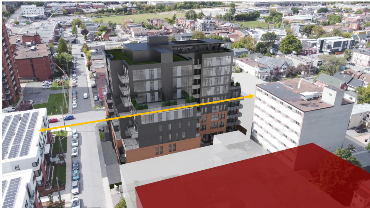
Figure 38: Views of the Proposed Redevelopment from the east showing transition.
