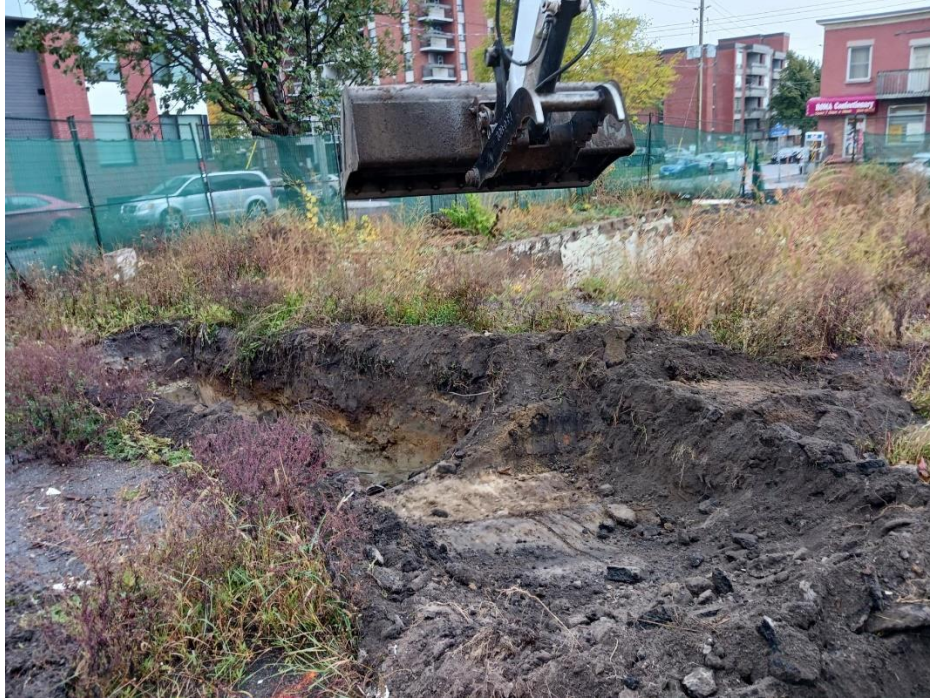
Image of excavation commencing
