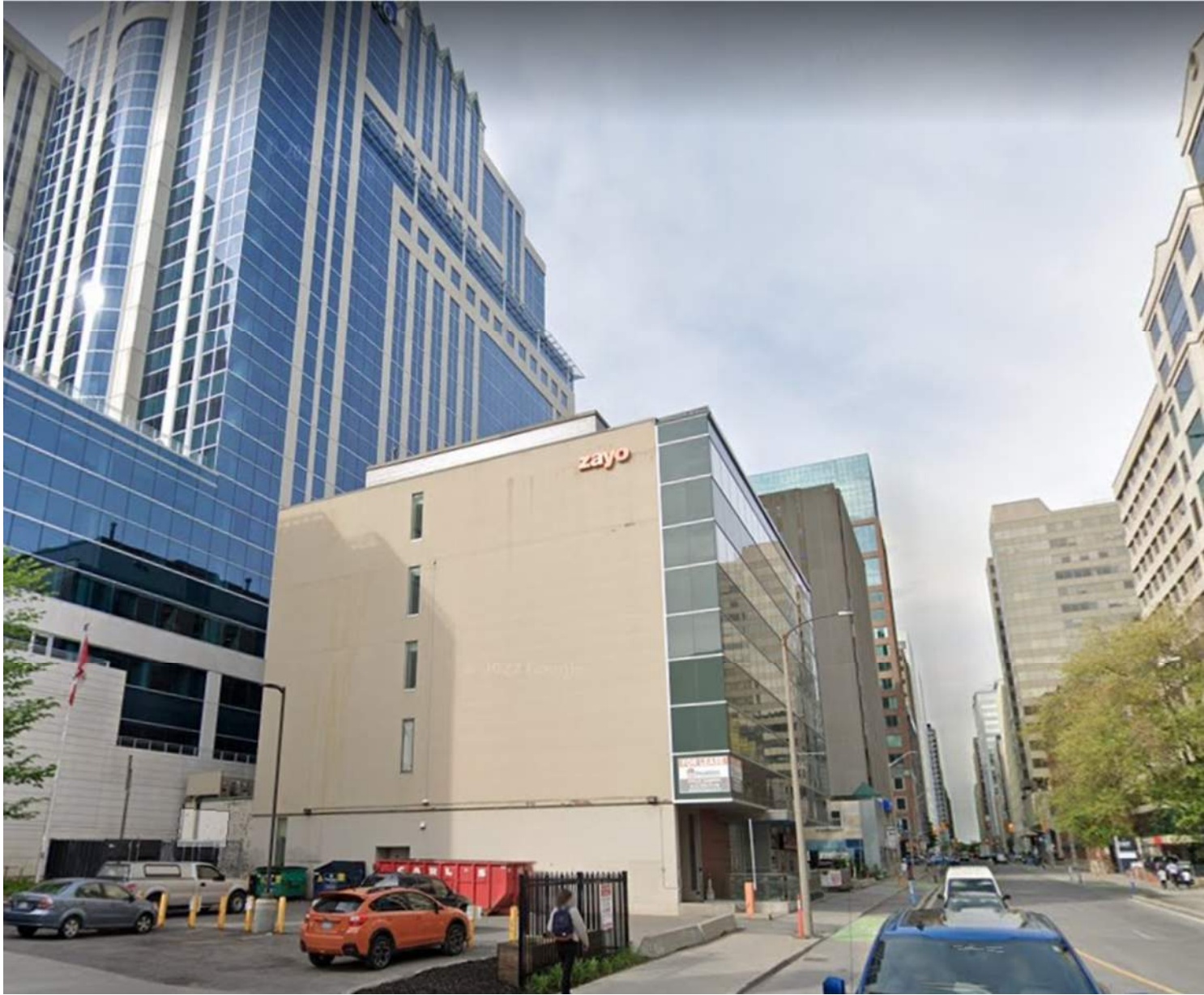
Subject Property, Looking West.
