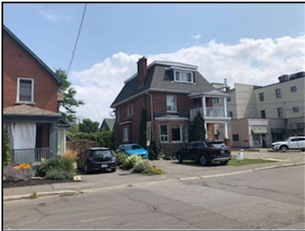
Photograph 2: Front view of 381 Winona Avenue looking southeast.
