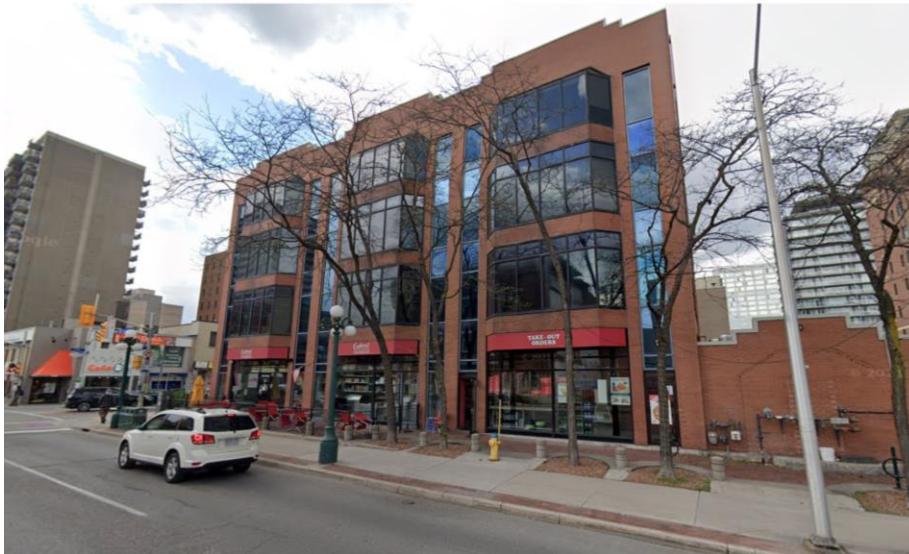
Figure 5: 350 Somerset at the corner of Bank is a 4-storey red brick that creates a bookend with the 2 1/2 storey buildings along Somerset Street. Source: Google Maps
