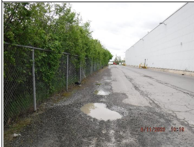
Photo 5: Existing Site Perimeter Fence
