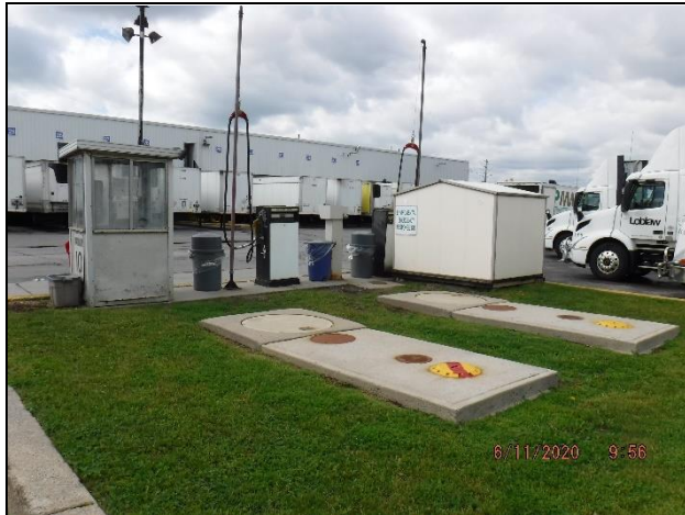
Photo 1: Existing Fuel Station
